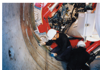
▲ On'chigawa-Higashi Trunk Line of Sewage System in Lower Stream of Neyagawa Basin, Sewage Pipe Construction Work (Lining Outer Diameter: 2,950 mm)
