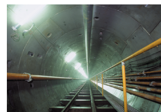
▲ Midorigaoka Rainwater Trunk Line of Sagami-hara City Public Drain Construction Work (Lining Outer Diameter: 3,120 mm)
